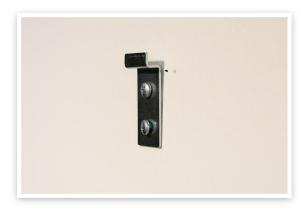
**STEP 2.**Recommend installing mounting hardware every 2 feet. Use a level to help maintain straight
